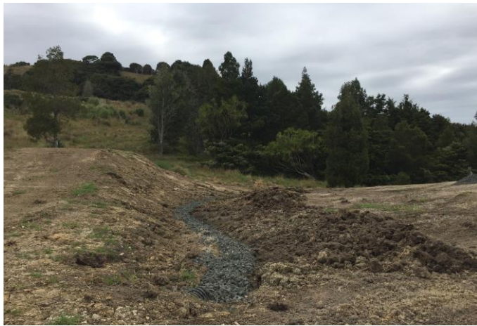
Photograph 7: Partially piped overland flow path in vicinity of new road
