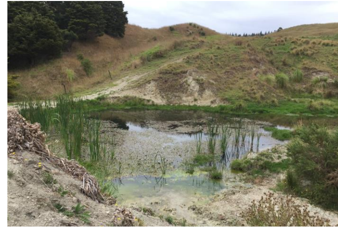
Photograph 10: Pond behind dam
