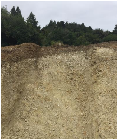
Photograph 5: Sample location SS01 (southern face of Bay 1 excavation)
