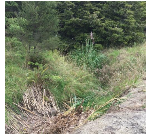
Photograph 8: Current head of central gully (down gradient from partially piped overland flow path)
