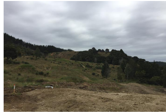
Photograph 6: Standing on future road looking northeast toward disused motocross track
